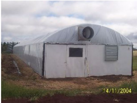
Figure 1: Tunnel rabbit shed with cooling system.
